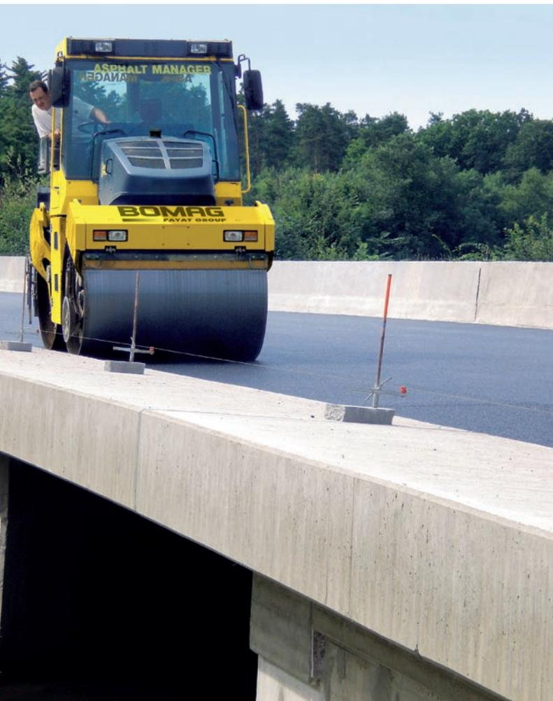
BOMAG offers the directed vibrator system, combined with BOMAG ASPHALT MANAGER, in both the 7t and 10t classes. The concept uses two counter-rotating, adjustable eccentric weights. If the weights point in the same direction, centrifugal forces increase whereas they are reduced as soon as the eccentric weights move into counter-directional positions.
